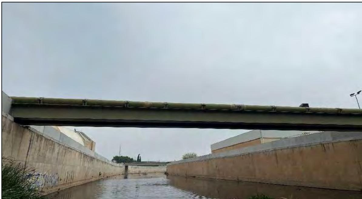
**Figura 3-14: Puente tuberías EDAR**
